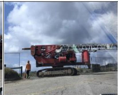
Drill rig entering property
